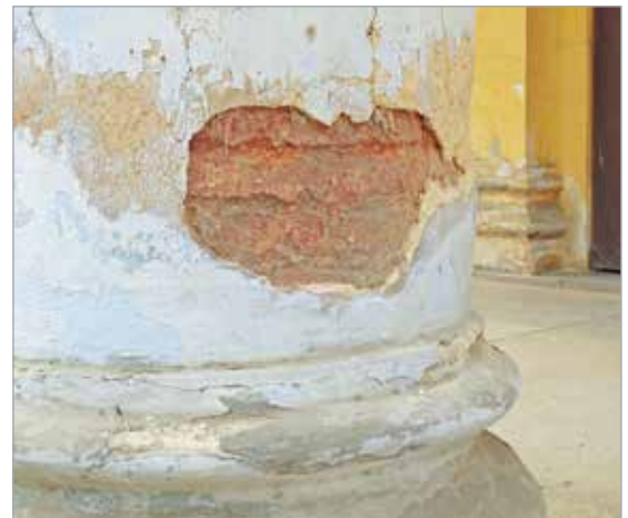
Pic 26: Exposed masonry on columns
