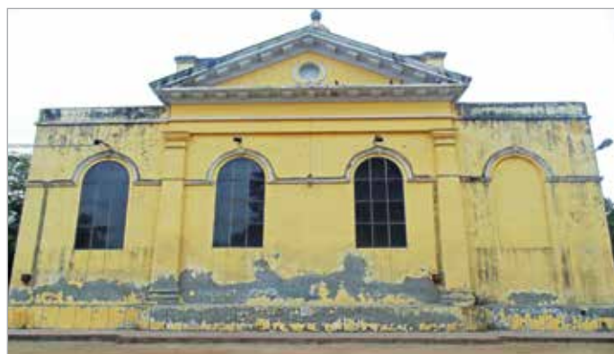
Pic 19: View of Eastern facade
