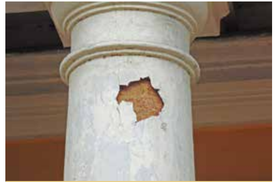
Pic 12: Exposed masonry on columns
