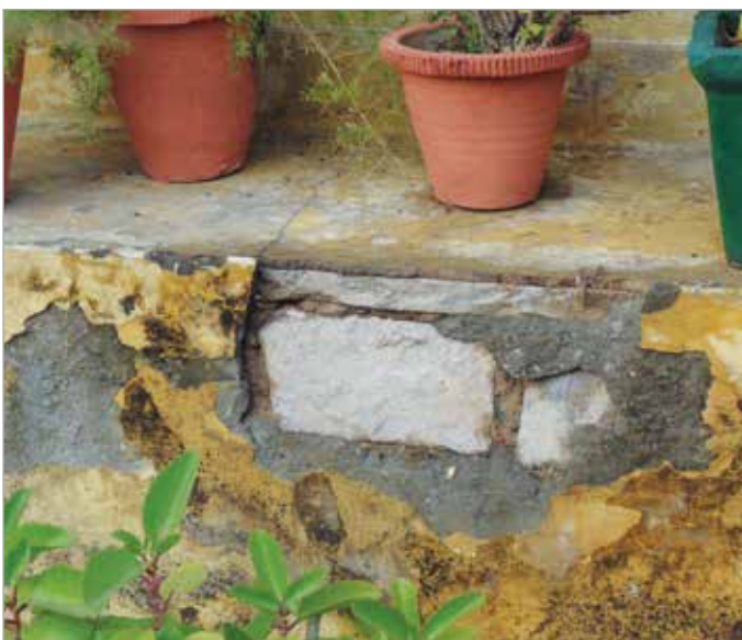
Pic 27: Exposed masonry at plinth level
